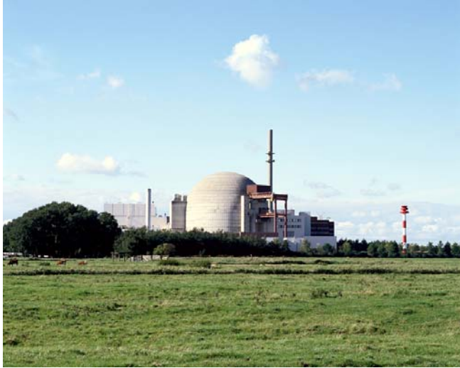
Nuclear power station Brokdorf (Germany)
